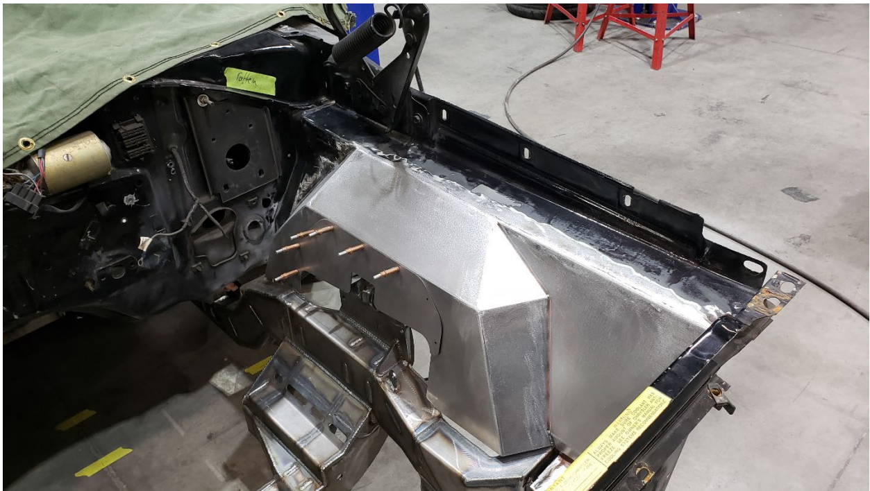
Figure 22: Installing the mounting plates
