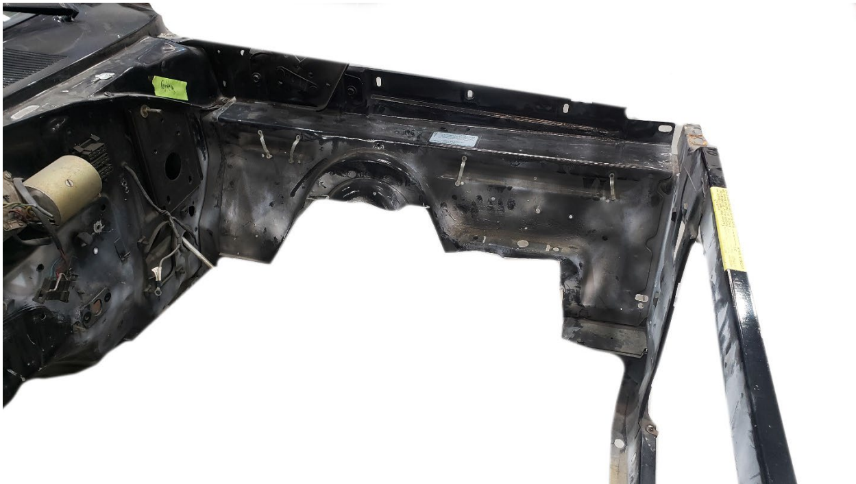
Figure 12: The floor of the driver's side of the vehicle
