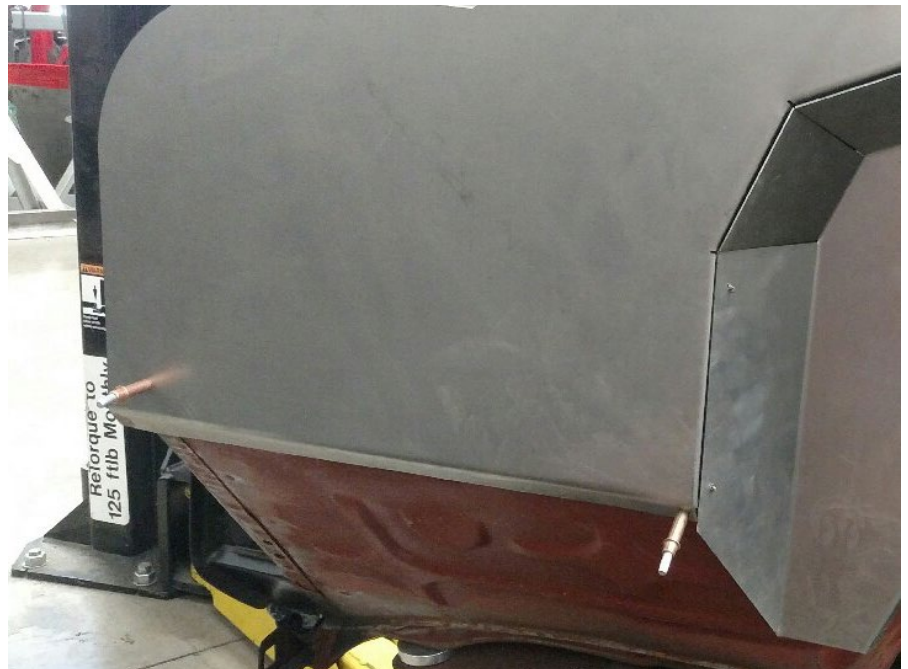
Figure 5: Bending the new firewall
