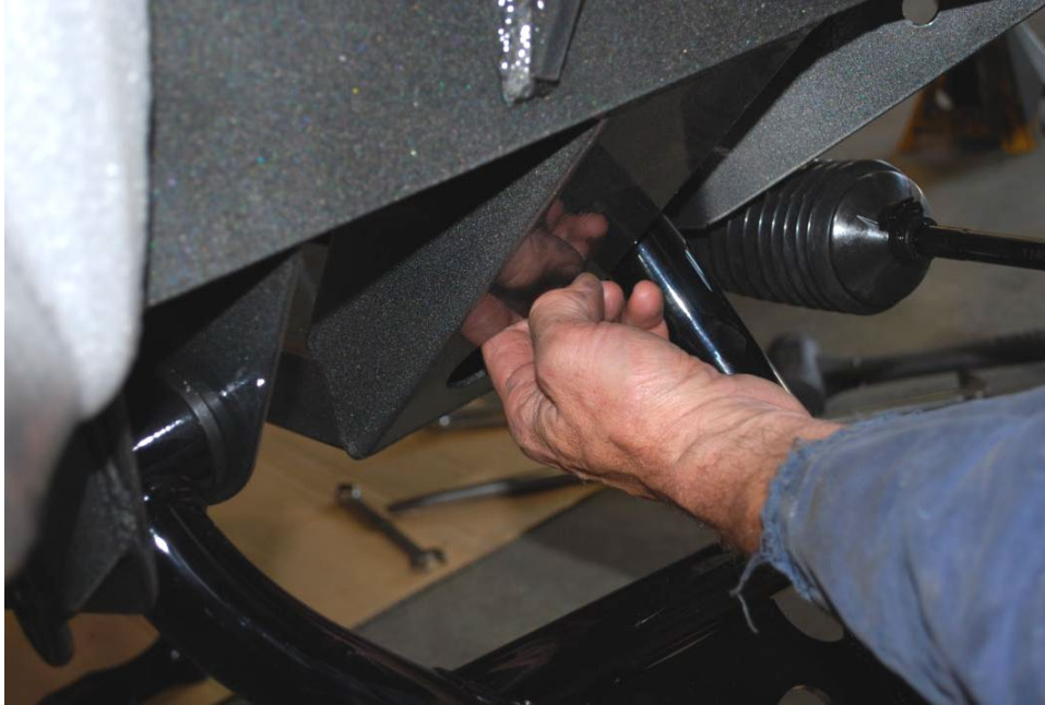
Figure 7: Where the lock nuts get installed
