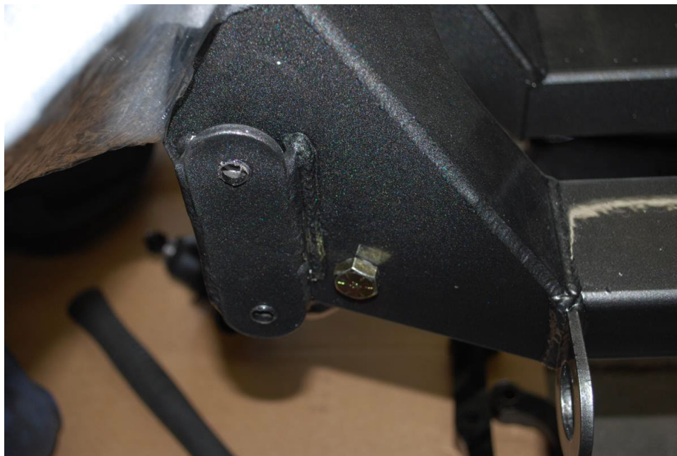
Figure 8: Location of where the sway bars will be bolted
