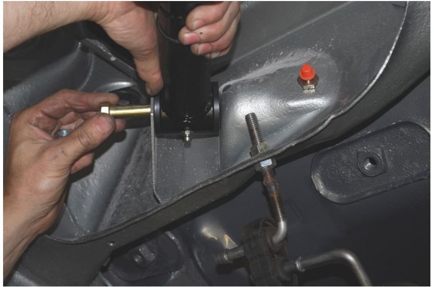
Figure 4: Installing the trailing arms
